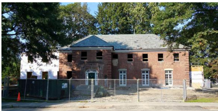
Above: Alfred Forbes '82 took this picture of the house under construction.
