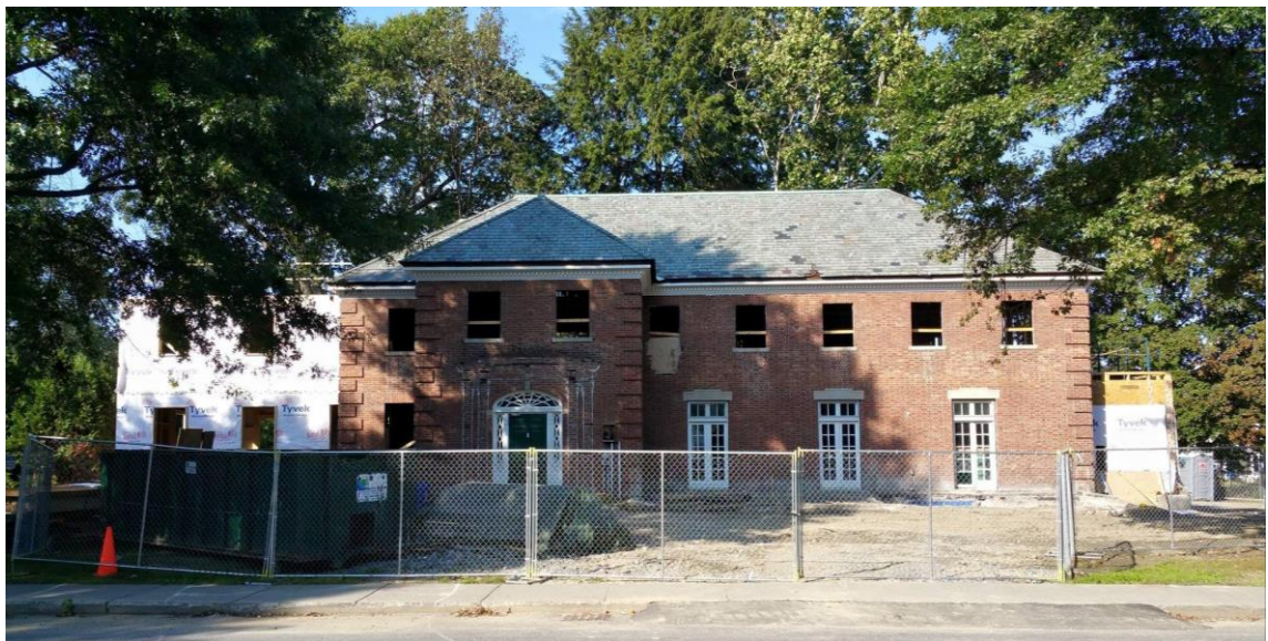
Alfred Forbes '82 took this picture of the house under construction.
